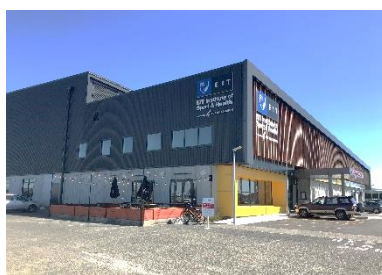
Mitre 10 Park Sports Hall, Hastings | Photo TCL
