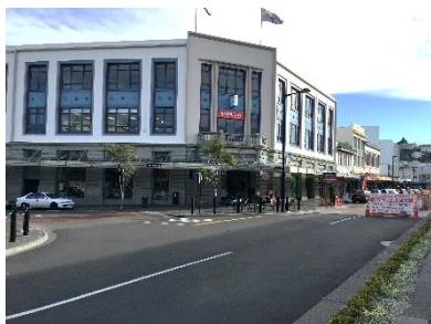
CPO Building, Napier | Photo TCL
