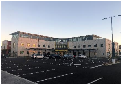
Hastings Health Centre | HHC Photo
