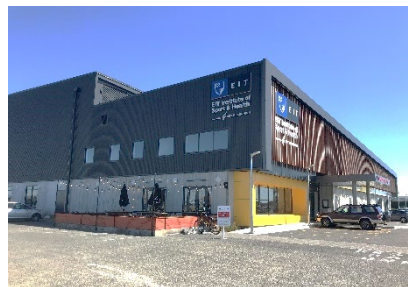
Mitre 10 Park Sports Hall, Hastings | TCL Photo
