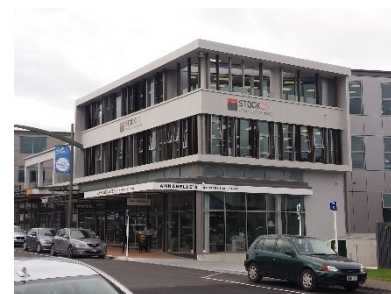
Village Exchange, Havelock North | T&Co Photo
